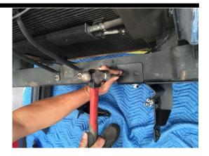
Using a Power drill, drill 11mm holes in the top surface and 13mm in the front.
